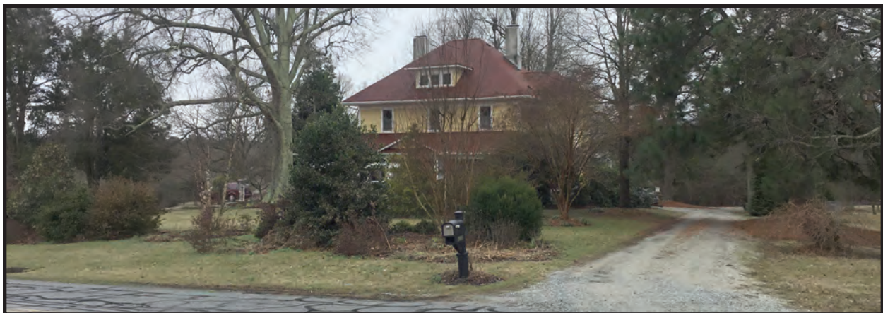
C. Facing West from Archdale Road
