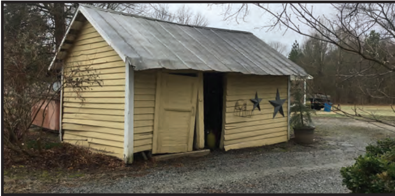
Figure 4.30. Bouldin House, Outbuildings
