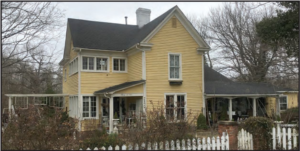
A. George Craven House (RD0818)
