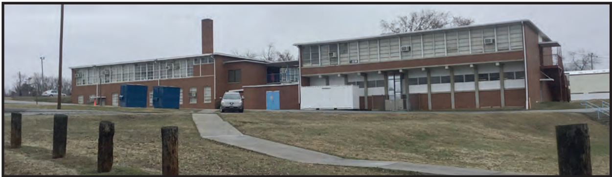
A. Classroom Building
