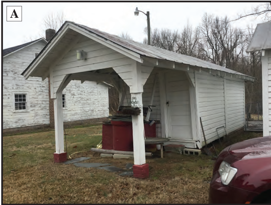
Figure 4.22. 3910 Archdale Road, Outbuildings
